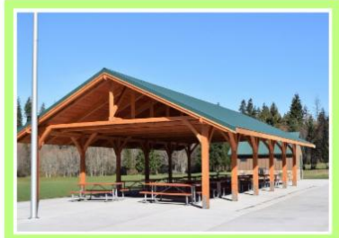
Gateway Park Pavilion
